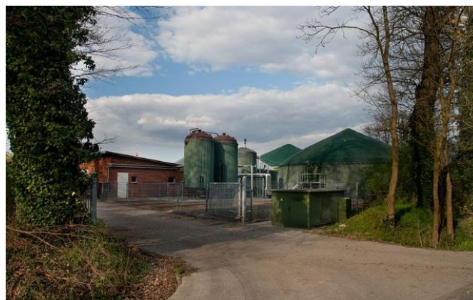
Figure 1: An anaerobic digestion plant in rural Germany
